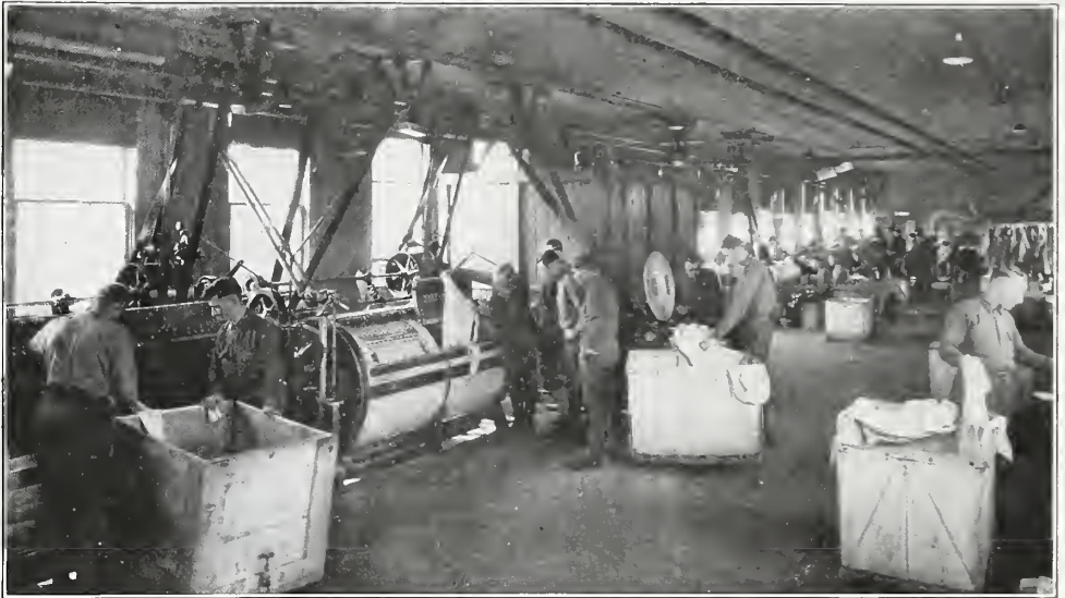
FIG. 81.—Laundry, Base Hospital, Camp Grant, Ill.
